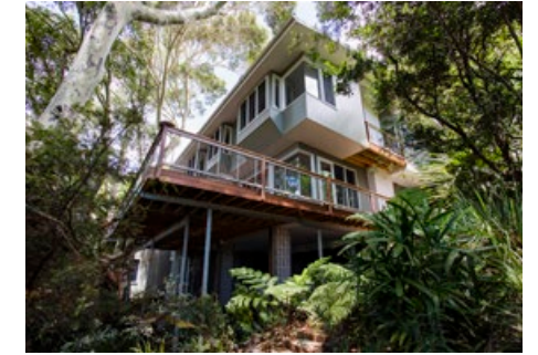
RESIDENTIAL ARCHITECTURE – HOUSES (NEW) CORYMBIA HUMAN SPACES BY JILL GLEAVE ARCHITECTURE PHOTOGRAPHER ST JOHN IMAGERY
