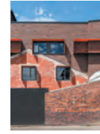
Thyne House Extension Project, Xsquared Architects with Robert Carroll & Associates
