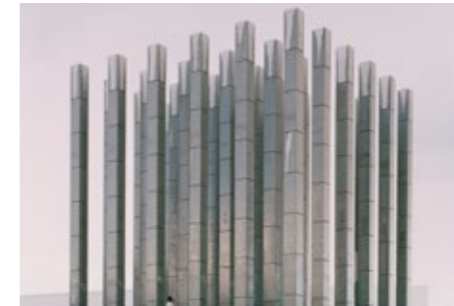
Small Project Architecture LESS Pezo Von Ellrichshausen, Oculus, and Molongio Photographer: Rory Gardner
