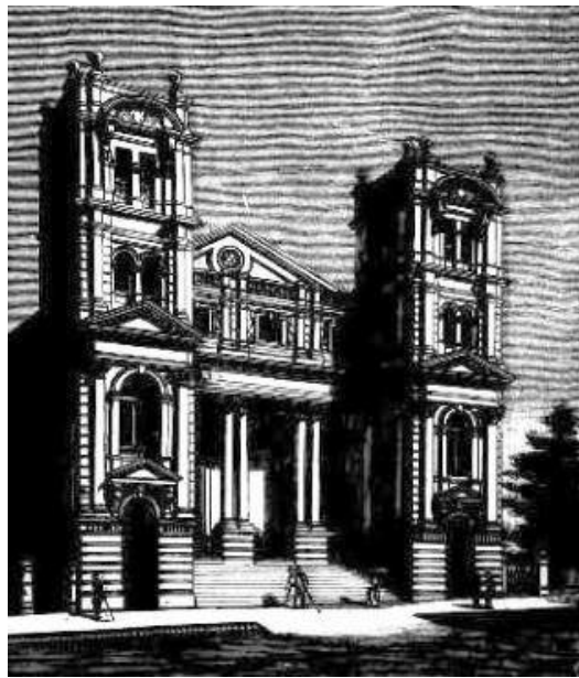
The Australian Church in Flinders Street Melbourne was demolished in the 1980s for the Harry Seidler designed Shell building opened in 1988 ( Australasian Sketcher , 27 January 1887, p.4)
