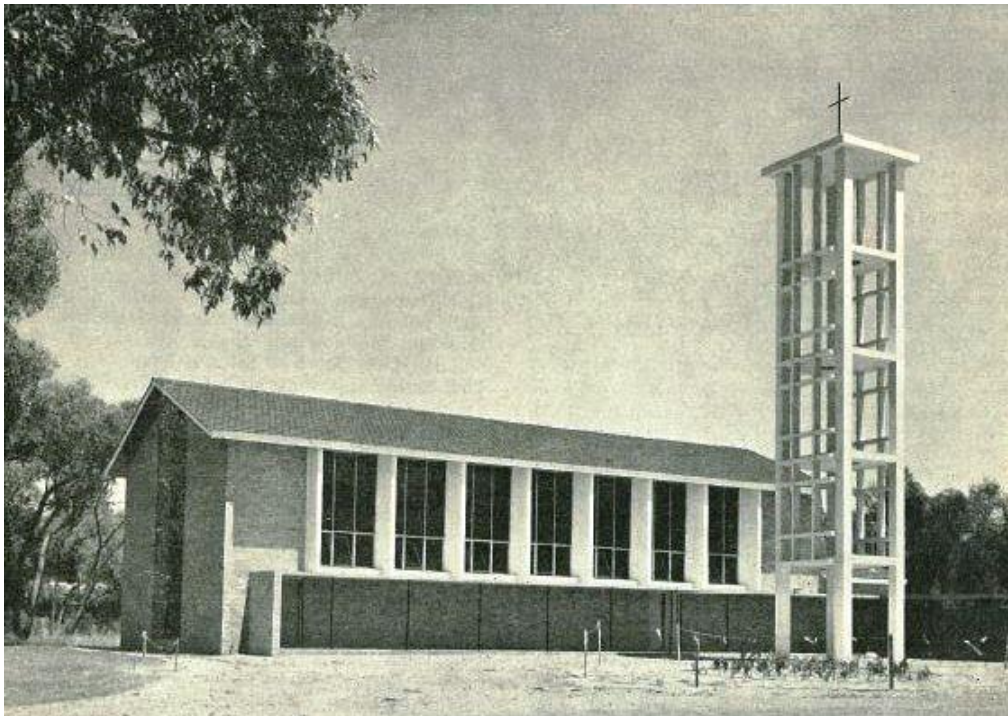
St Thomas More Chapel at UWA of 1954 ( The Architect WA , December 1957, p.29)
