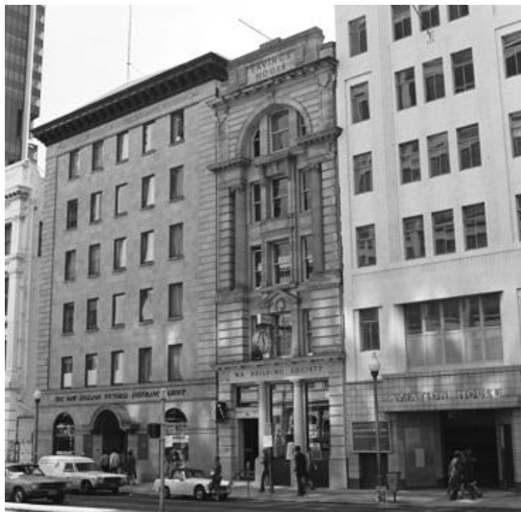
Now demolished, Hawkins' first project in Perth was the Victoria Insurance Company Building at 98-102 St George's Terrace (at left of photo), completed in early 1929 (SLWA 360986PD)
