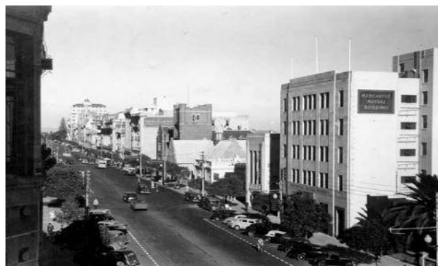
Sketch for Mercantile Mutual Building; and (right of photo) at 179 St George's Terrace, Perth in 1947 ( The West Australian , 30 October 1937, p.8; SLWA 000212D).
