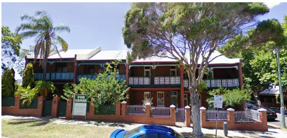
Four 2-storey cottages cnr Monger & Lindsay Streets Perth of 1916 (Google 2014)
