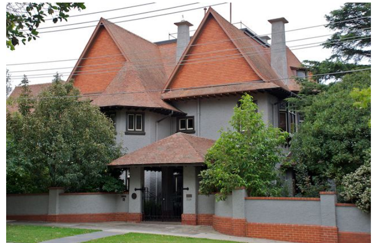
View of south west corner 2010, photo by Peter Johnson
