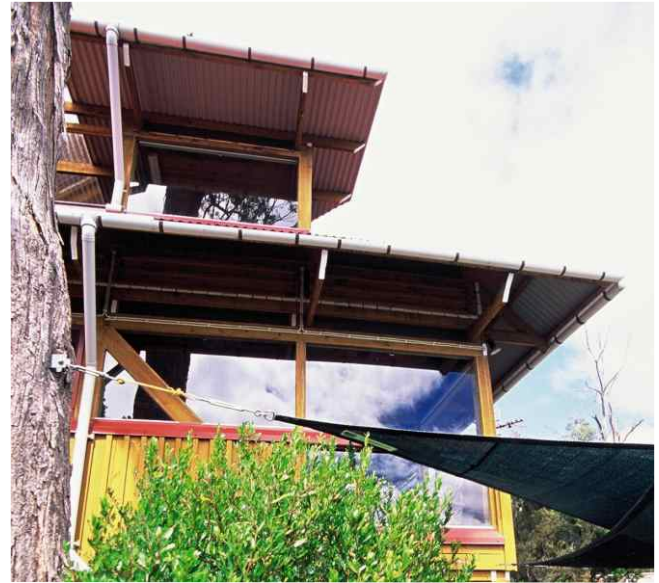
Characteristic timber framed post and beam construction
