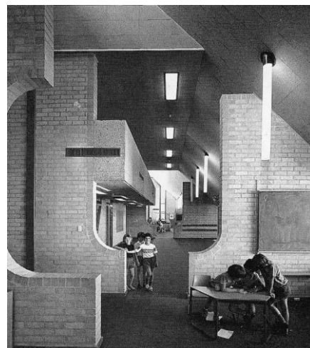
Interior of Primary & Infants School with library balcony. (Source: Aust. Architecture Since 1960; Jennifer Taylor, RAIA)
