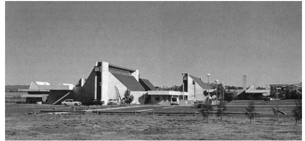
Primary & Infants School & Neighbourhood Healthcentre. (Source: Aust. Architecture Since 1960; Jennifer Taylor, RAIA)
